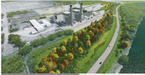
NAPANEE GENERATING STATION
