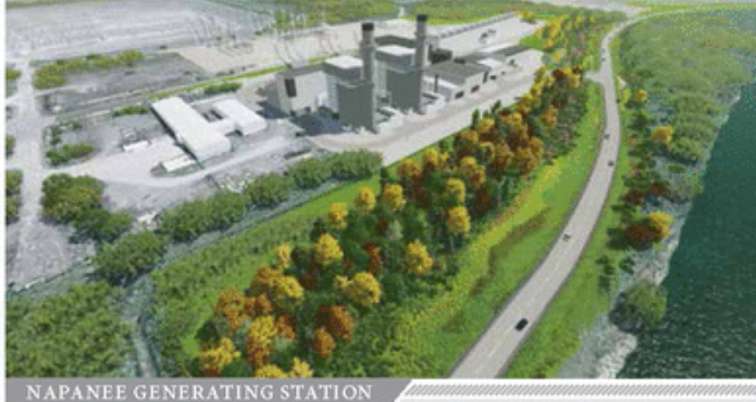
NAPANEE GENERATING STATION
